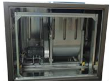
Figure 13. Electric Heater in AHU
